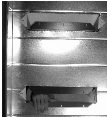
figure 2.3b - Unfold the ducting flairs completely to sandwich the return air plenum between the ducting flair and the filtration unit.
