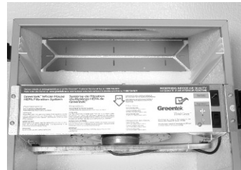
figure 2.2c -The unit should look like this when the foam piece is removed.
