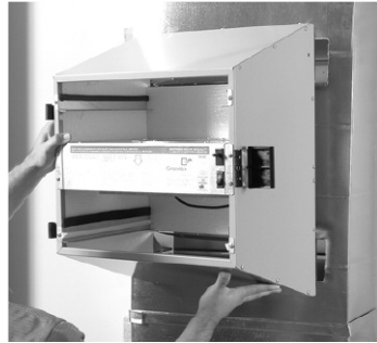
figure 2.3a - Align unit into place.
